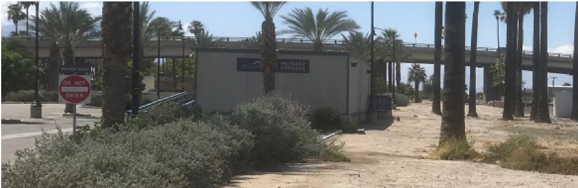
Union Pacific Railroad Corridor at Jackson Street
