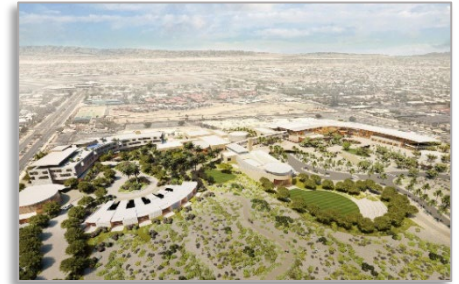
Aerial Site View
