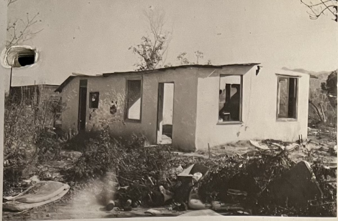
Structure on Blk. 39 10/26/65 da/ar
