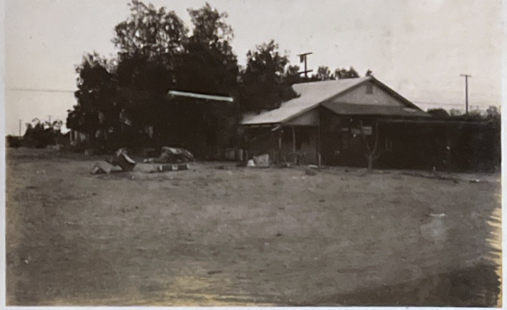
Structure on Blk. 87 Southeast View 11/2/65 da
