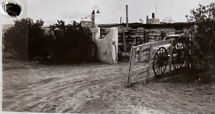
Structure on Blk. 231 Northeast View 11/24/65 da
